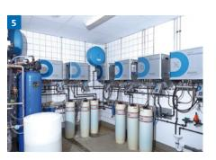
tank. By deploying this standardised process water, Heidelberg ensures that the ink/water balance for the ink in the machines remains stable, and that toning, roller glazing or setoff does not occur. The water has a constant quality, with a pH value between 4.8 and 5.5 and a hydrogen carbonate content of less than 150 mg/l.
