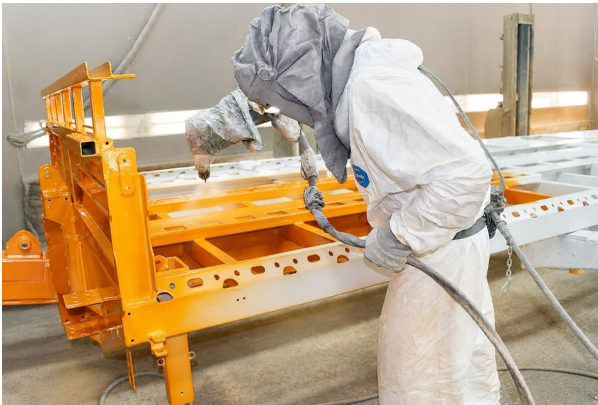
Duplex coating: hot-dip galvanising + paint finish = maximum service life
