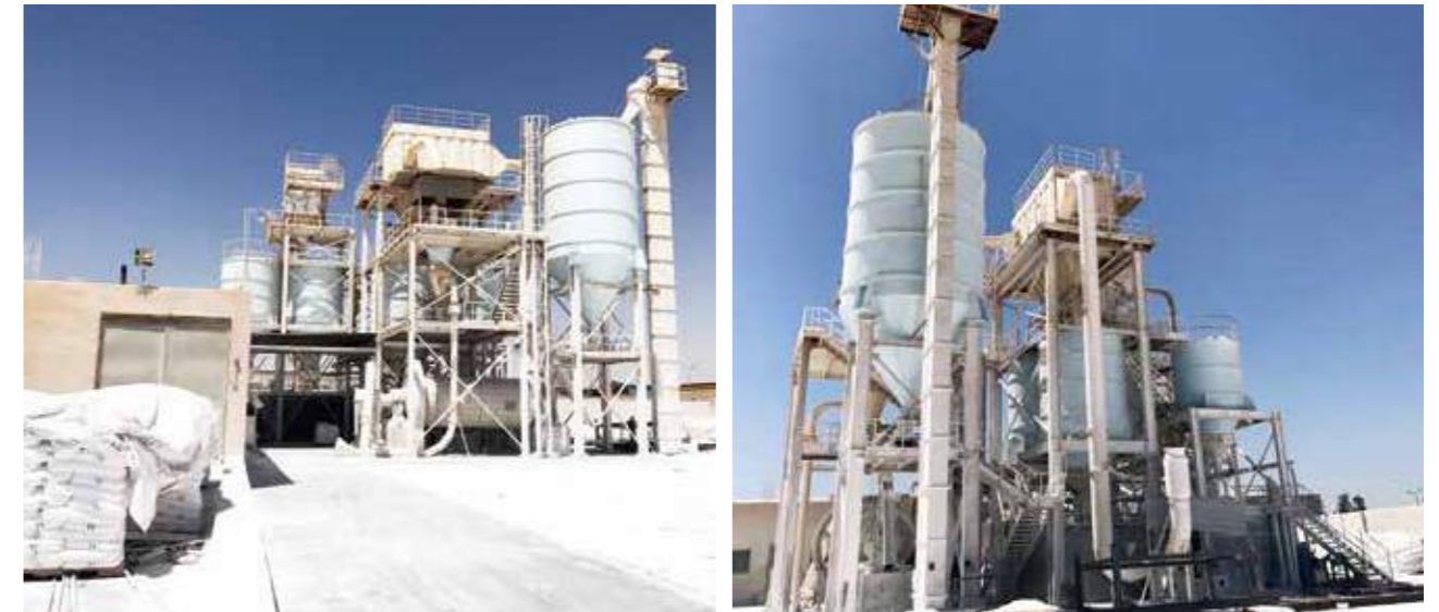
40,000tons/Year Calcium Carbonate Ball Mill Plant and Coating Plant In Egypt, Year 2015 (Φ2.2*5.5m Ball Mill)
