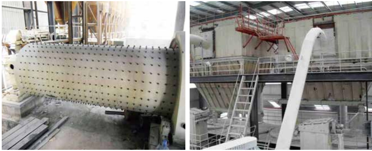
100,000tons/Year Kaolin ball mill plant in China, year 2024 (Φ3.8*11.0m Ball Mill)
