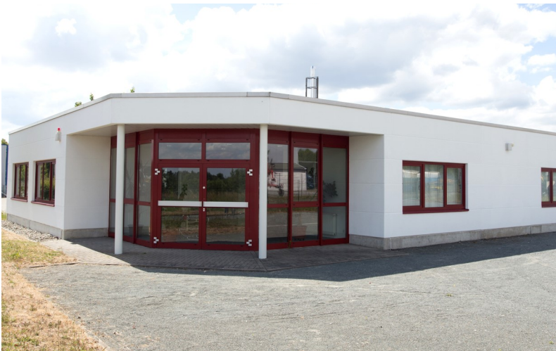
Schulungsgebäude FIMRO / training centre at FIMRO
