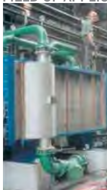
Liquid/liquid energy recovery
