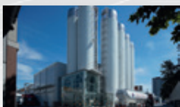
Silo and discharge systems
