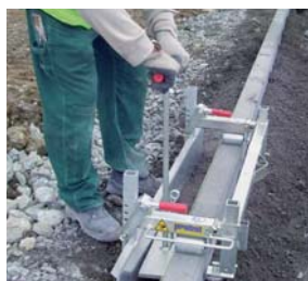
Slipform for Concrete Kerb Backfill GR-150
