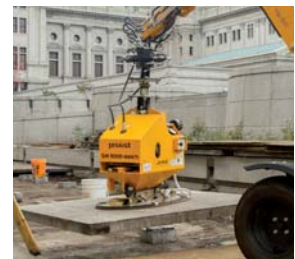
VM with Vacuum Attachments SH-1000-MINI-H
