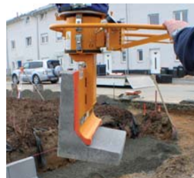
Special suction plate for angular concrete products
