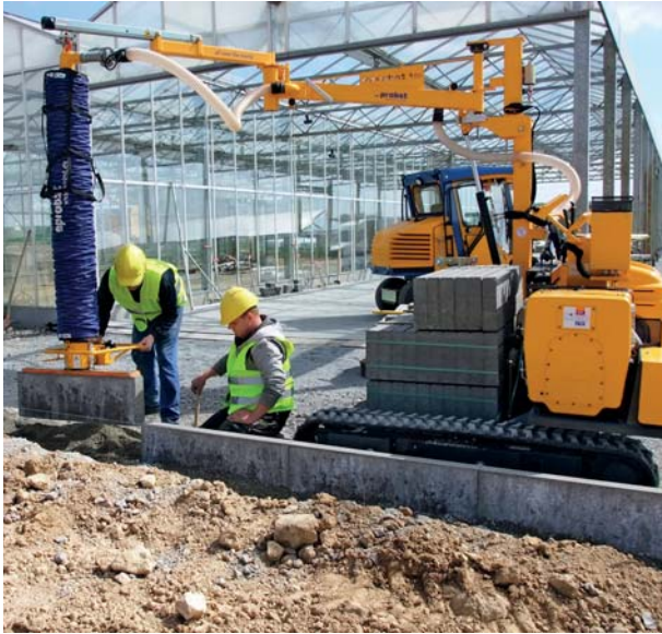
TRANSMOBIL TM Installation Carrier installing kerbs
