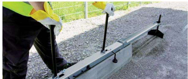
BOBPLAN BP Pulling aid for the concrete subgrade
