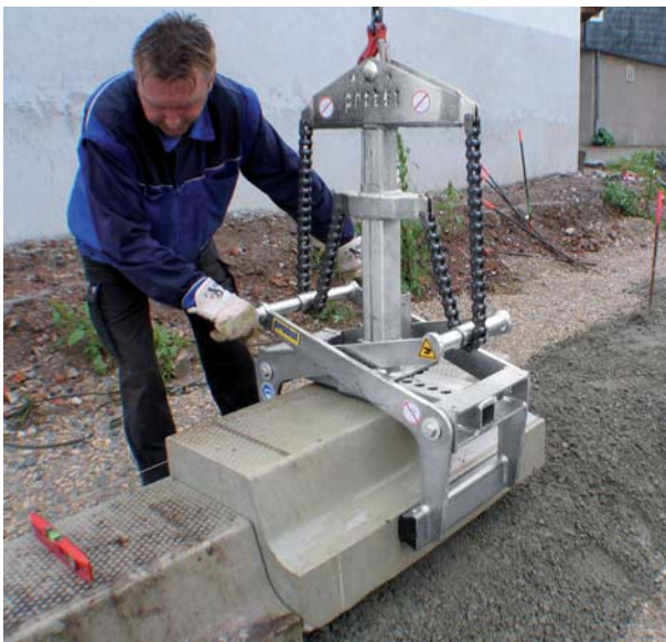
Grab for Prefabricated Concrete Products FTZ-UNI-15
