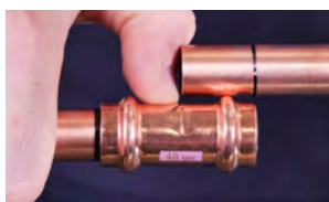
7b. Check the depth mark
