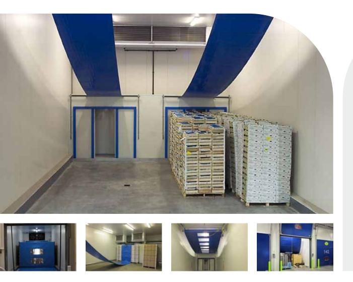
he Tarp is manufactured from Trevira fabric with PVC coating and has fibreglass reinforcement bars to resist air pressure. The Tarp is fixed onto the suction wall with special guide tracks and rollers for adjustment to different pallet heights. This pressure roller secures the Tarp to follow the pallets and guides it to cover the pallets completely airtight. We advise placing our integrated and depressible foam buffers (100x100) on the suction wall to prevent air by-pass behind the pallets.
