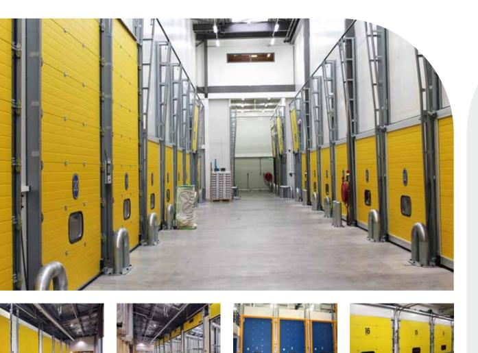
S uited for storage rooms, fruit ripening chambers (including tropical fruit and in particular bananas). The door consists of sections. Tracks are selfsupporting and (depending on the rail system) the door leaf is guided horizontally, vertically or following the roof pitch. The spring systems are pre-assembled with powder-coated springs. Cable break bottom fixtures are standard supply. The sections are structured according
