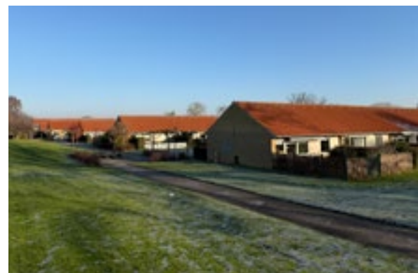
Maerskgaarden residential community has replaced gas boilers with a heat pump.
