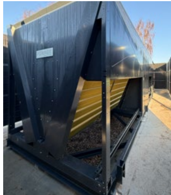
Close-coupled heat pump and V-shape evaporator (energy collectors) installed inside a sound enclosure.
