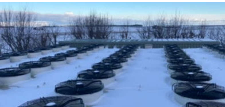
The FENdefrost system ensures reliable operation of the evaporators even in snow and frosty weather.
