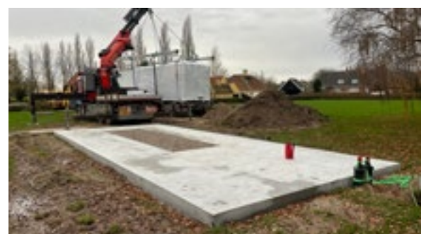
Delivery on site. The close-coupled heat pump is here installed on a concrete foundation.
