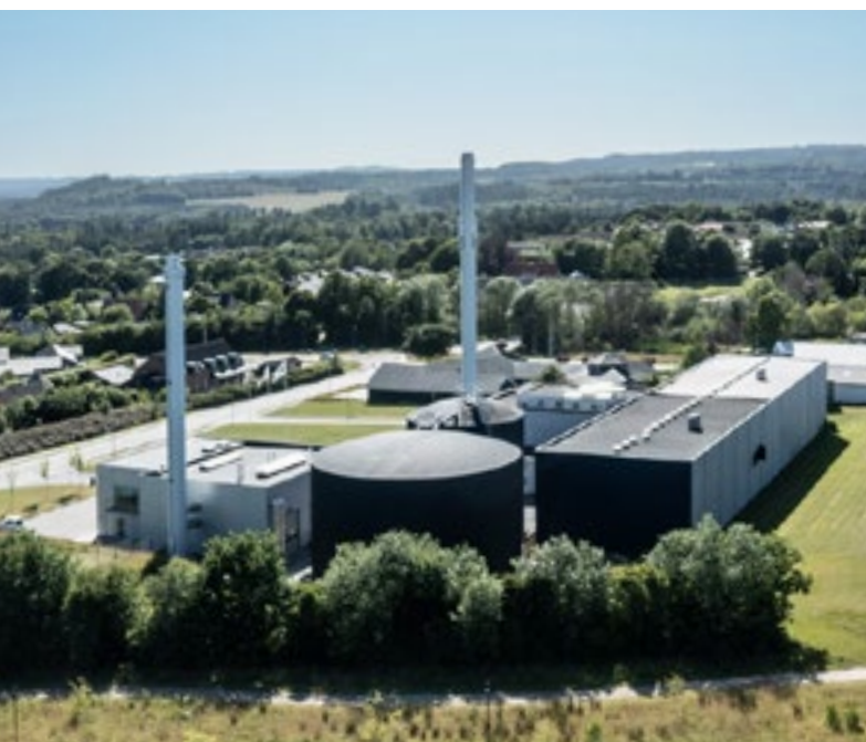
Original site expanded with accumulation tanks
