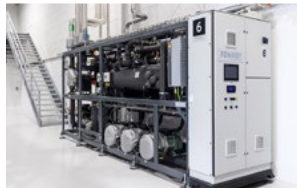
C-300 chiller unit (with heat recovery) for cooling of machine room and transformer room
