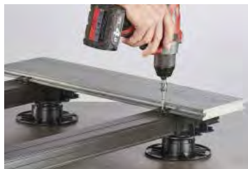
3. Mount the mounting bracket
