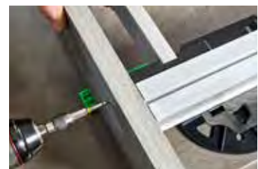
2: Fastening panels with adapter for transverse bracing see p. 48–49
