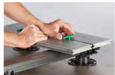
4. Use the correct installation aid
