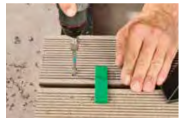
4. Screw the patio deck in place
