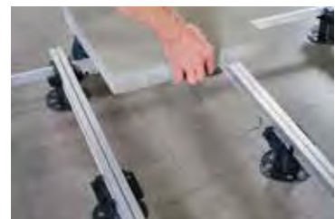
4. Insert the slabs
