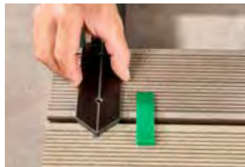
1. Apply drilling template
