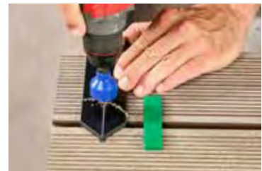
2. Mark the drill holes with a drill
