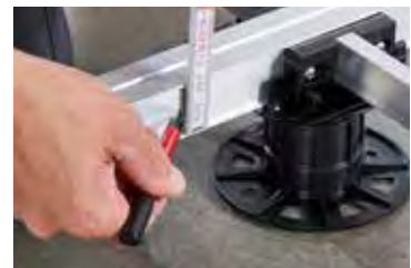
2. Drill holes (6 mm) in the centre of the substructure
