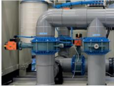
A  $CO_2$  adsorber, also known as a scrubber, removes carbon dioxide from cold stores, along with a small portion of the harmful ethylene present. The  $CO_2$  adsorber contains active carbon, which has the characteristic of adsorbing  $CO_2$  molecules (binding them to it). By efficiently transporting the air from the cold store, passing it over the active carbon and returning it to the cold store, the  $CO_2$  is effectively removed from the air in the store.
