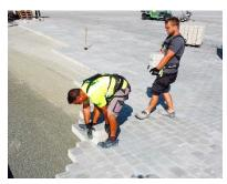
The BionicBack exoskeleton assists in lifting and carrying heavy objects such as planting soil, stones, paving stones, and building materials.
