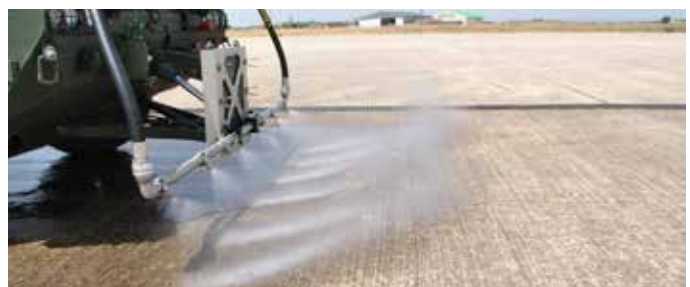
Decontamination of road sections
