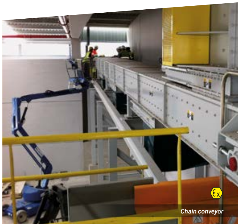
Central section of Redler in stainless steel
