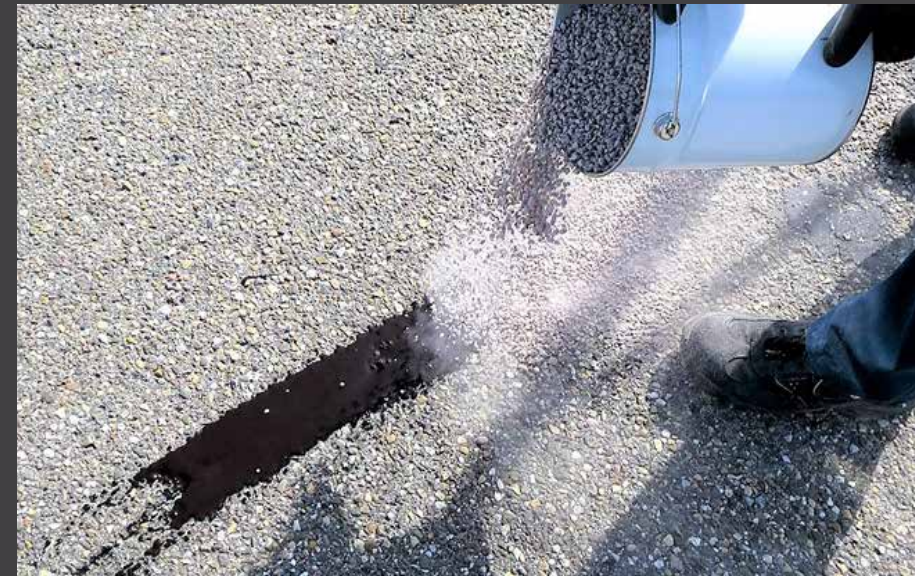
Crack Repair
