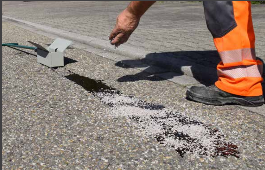
Crack Repair
