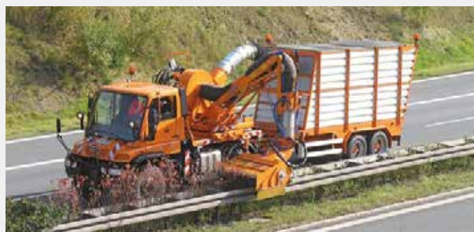
Cutting vegetation above a crash barrier with HSK 1200
