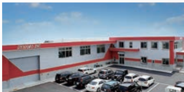
■ Main Office Dynamo, Inc.
