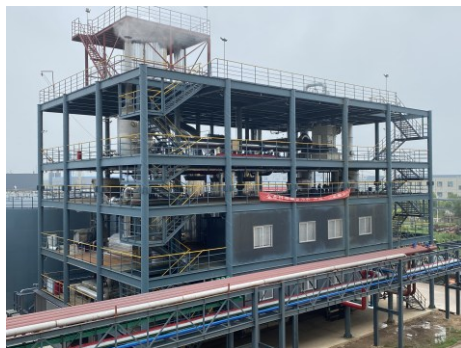
System integration installation
