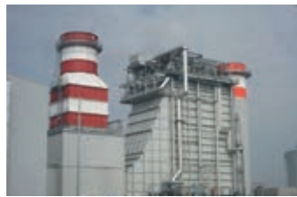
Gama Generation Facility Ireland
