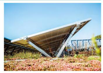
photovoltaic panels through the shading and cooling effect they have on the roof, thus reducing the temperature of the solar panels, increasing their efficiency. Due to the raised panels, roof maintenance is facilitated and specific microclimates are created with variable temperatures and humidity in the areas shaded by the panels, which favor a diverse range of plant and insect species.
