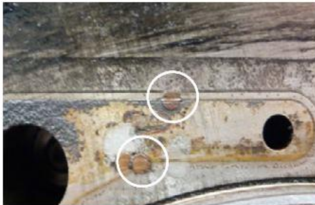
Faults in base material - epoxy repair
