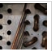
Internal Re-heat Coil
