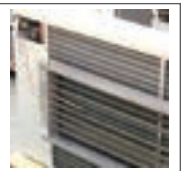
External re-heat coil
