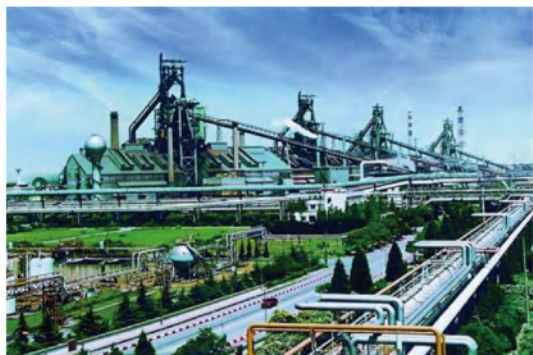
China Baowu Steel Group Co., Ltd.
