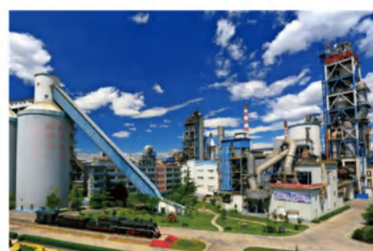
Tangshan Jidong Cement Co., Ltd.
