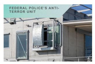
A true-to-original aircraft door is integrated into the modern training center of the Austrian special forces unit. It enables realistic training for aviation-specific operational scenarios.
