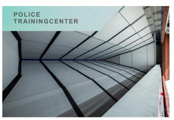
Funnel-type bullet trap with an automatic discharge system, engineered for official service weapons and standard calibers up to 20,000 joules.
