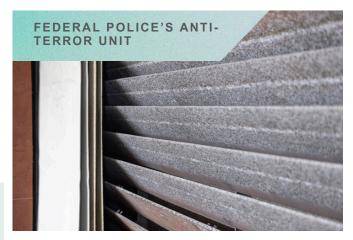
State-of-the-art steel lamella bullet trap with an automatic discharge system, specifically designed for use with official service weapons and ammunition.
