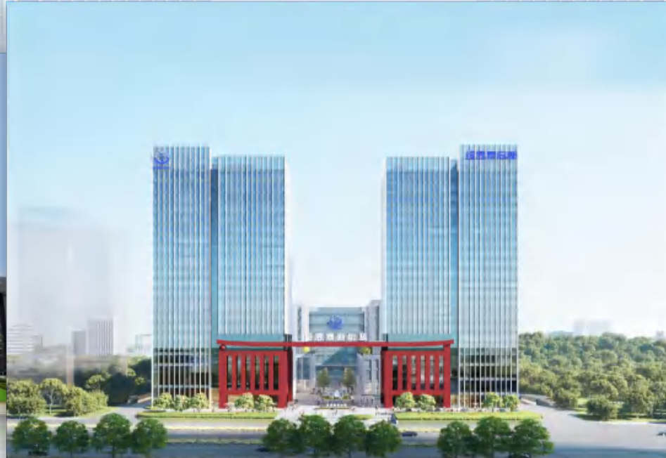
Third production base (Under Construction)
