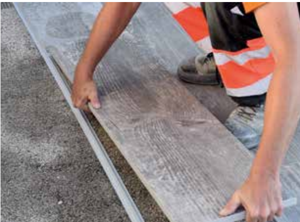
No rocking due to continuous support of the slab edge.
