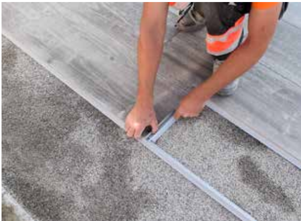
The cross profiles can be slid under the slab at a later stage.
