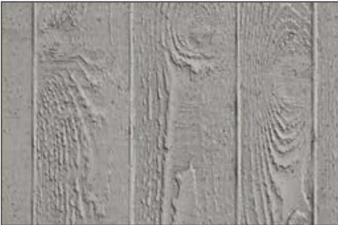
122 Brettschalung | timber formwork
