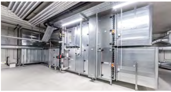
PERFECTION CANNOT BE TAKEN FOR GRANTED
