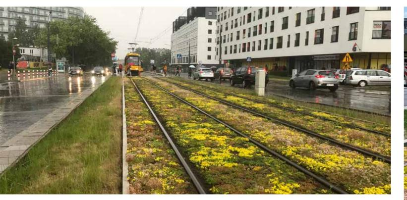
Sedum-mix blankets are easy to apply. The vegetation remains low, so that trams and trains can pass over them without any problems and the view of road users is not restricted. In addition, Sempergreen's green groundcover systems are lowmaintenance.
