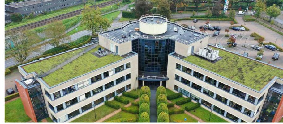
With these systems, rain can be collected where it falls first: on the roof! Relatively lightweight and suitable for sloping roofs, the Detention roof can be used on renovation projects. A Retention roof is a versatile solution for new construction projects, and can be combined with solar panels and biodiverse vegetation blankets, for example.
