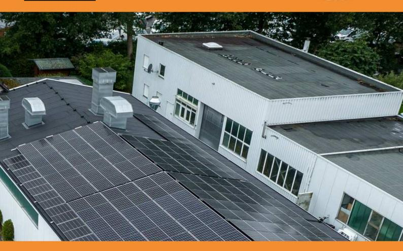
Sustainability is important to us and that's why we have 65 photovoltaic modules, with one Power of 57KwP installed on our roof. This means we reduce our energy consumption from fossil fuels by around 50%.
