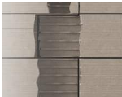
Make a wall niche to install the siphon and the condensate
