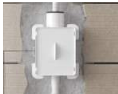
Protect the siphon by applying the protection cover
