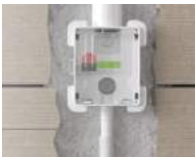
Plaster the wall niche
