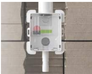
Put the siphon into the wall niche
