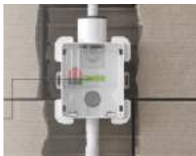
Connect the pipes. Check horizontal level
