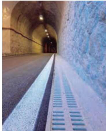
Castillon Tunnel. France
