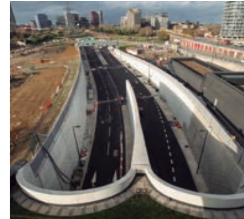
Silvertown Tunnel. United Kingdom
