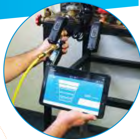
MEASURE EVACUATION WITH THE SI-RV3 VACUUM PROBE
