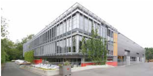
The development and sales centre with assembly halls of Müthing GmbH & Co KG Soest.
