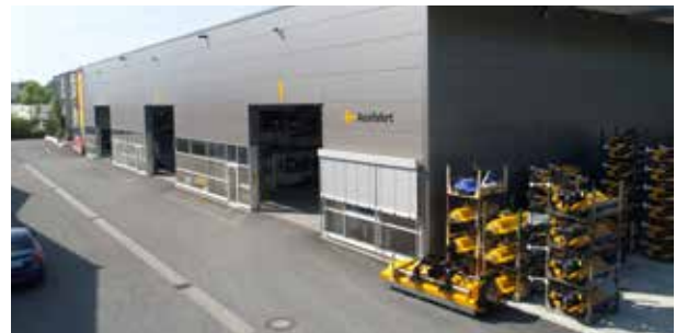
The assembly hall at the Soest location - Technology in perfection.
