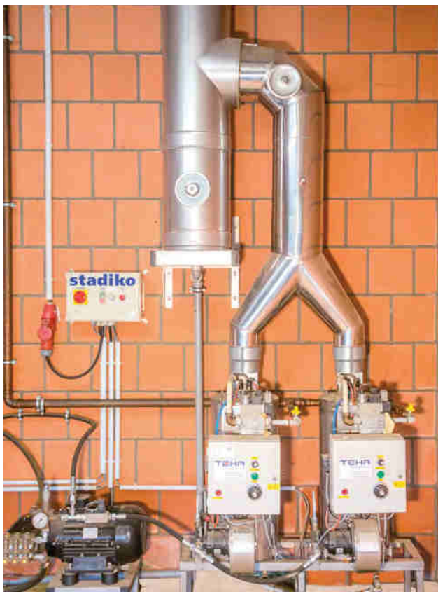
Stationary HD 7.5/30-130 with a double burner chamber
