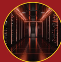
Cloud & Data Center
