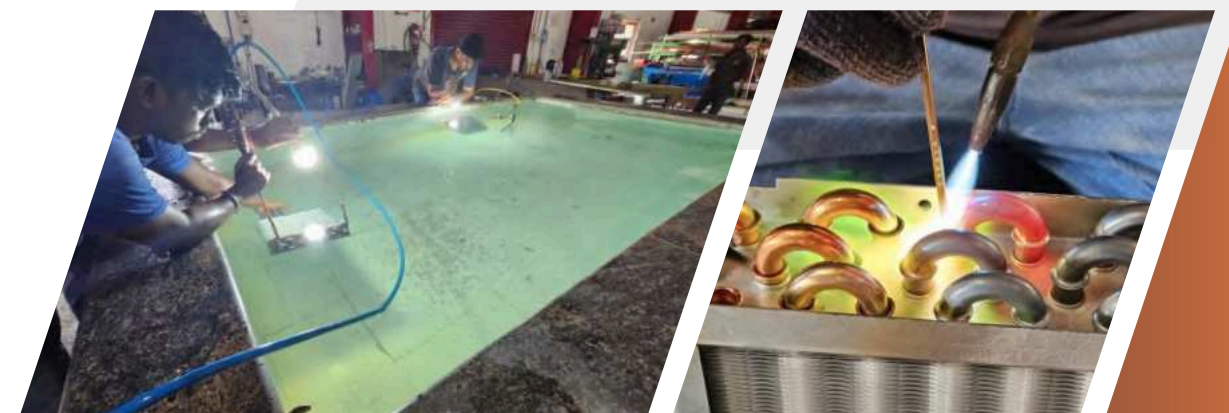
LEAK TESTING & BRAZING SETUP
