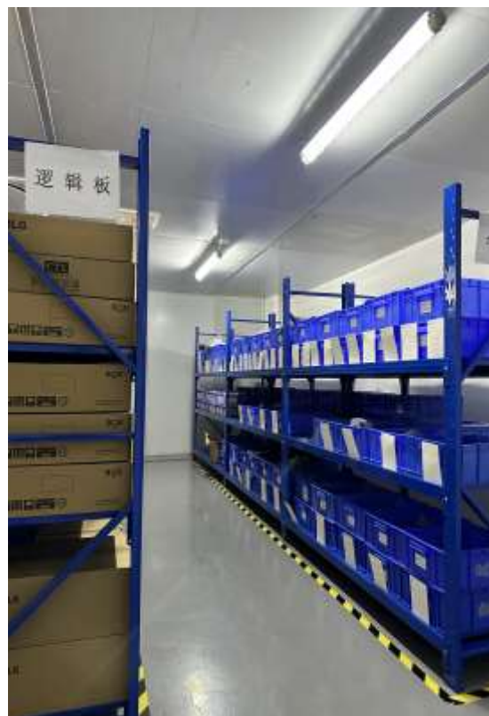
Warehouse Electrical Material
