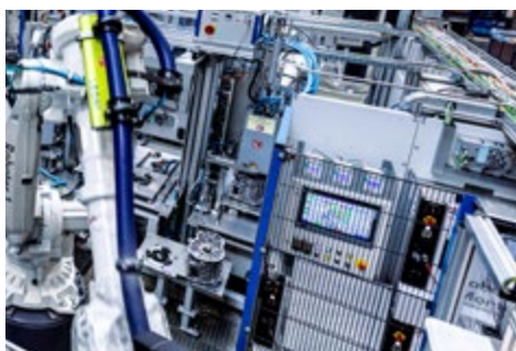
VA: Joining of the bearing bush incl. position and temperature monitoring
