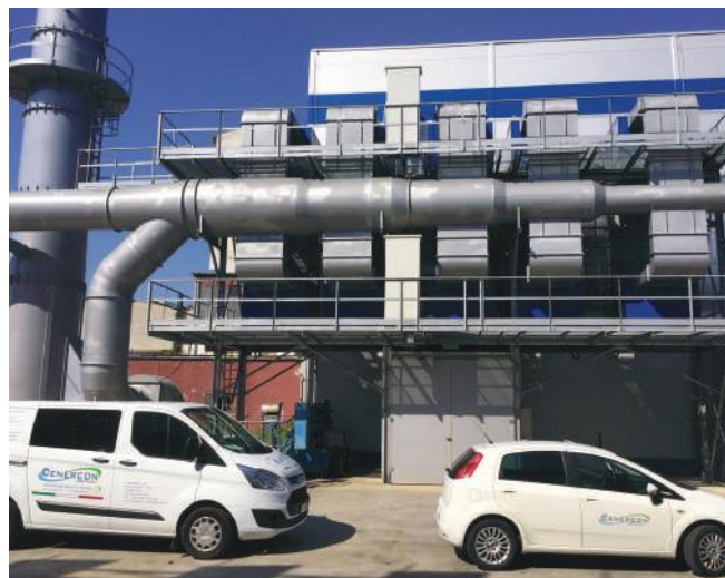
ENERPROG centralized suction and filtration system in 10 modules for a total suctioned flow of 150,000 m 3 /h for 19 presses - Slovakia
