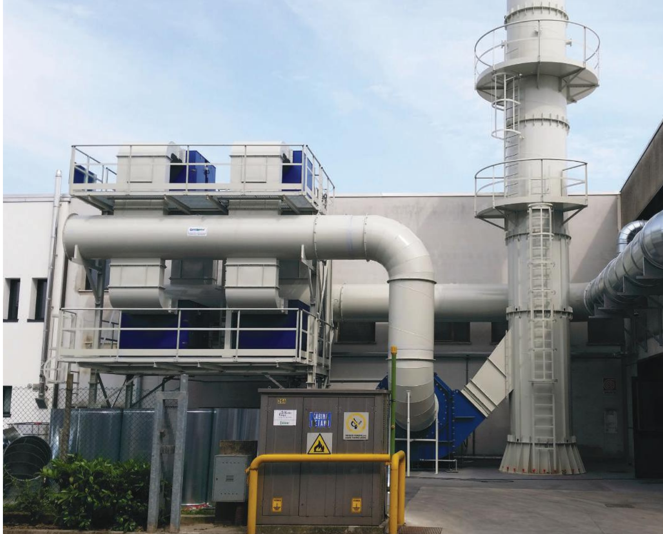
ENERPROG centralized suction and filtration system in 4 modules dedicated to 7 presses - Italy
