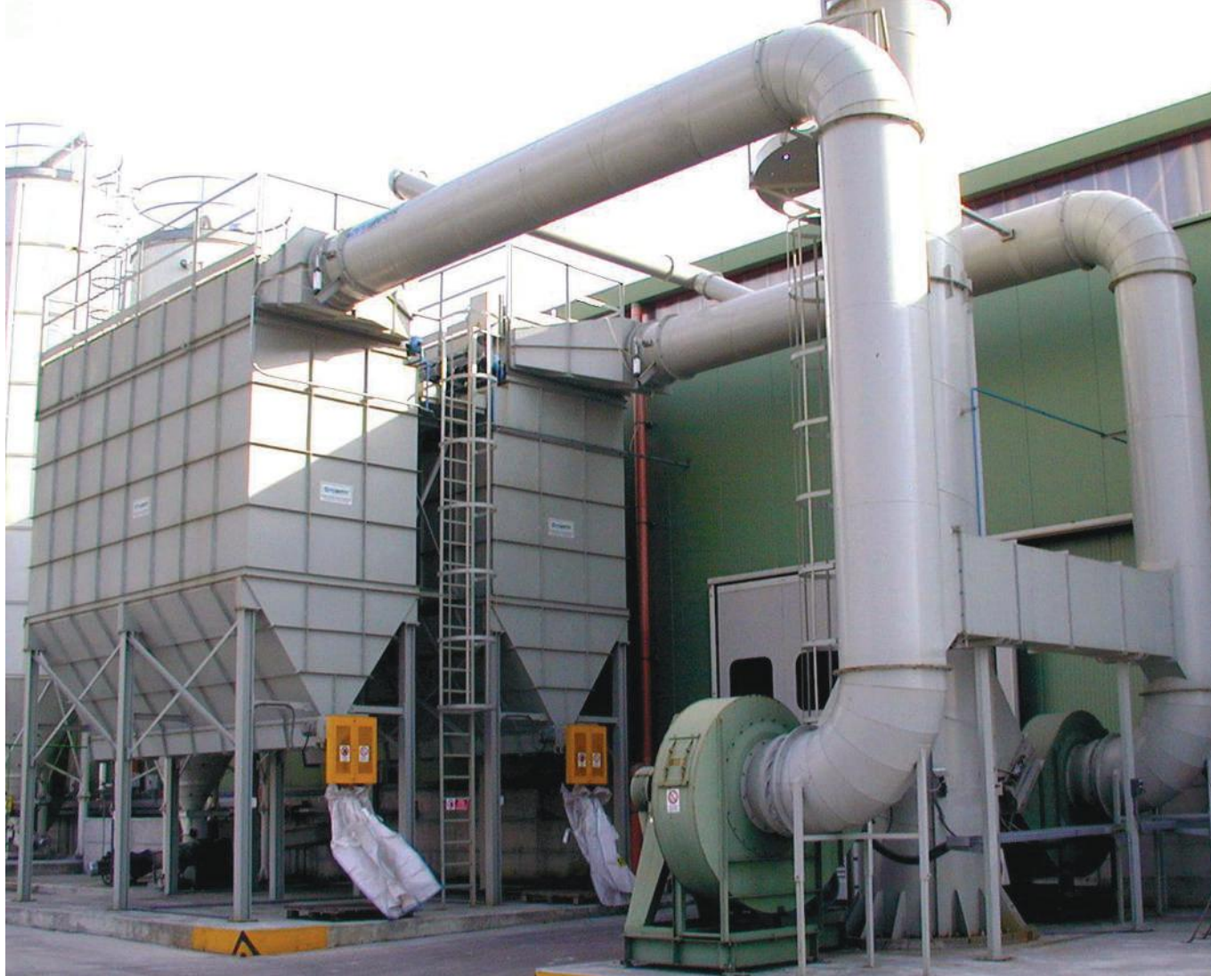
■ Suction and filtration system for dusts - Italy
