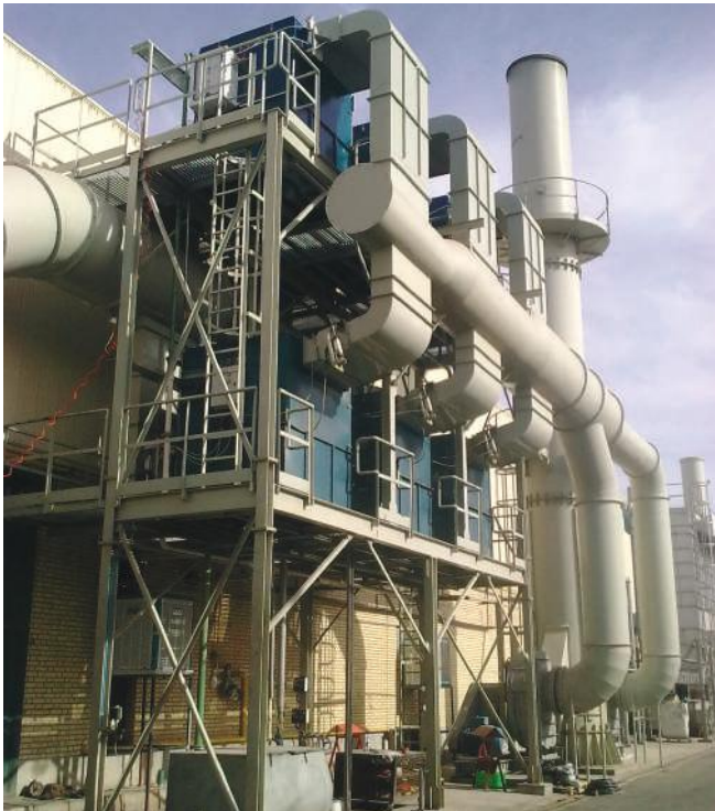
ENERPROG centralized intake and filtration system in 6 modules dedicated to 4 large tonnage presses - Iran
