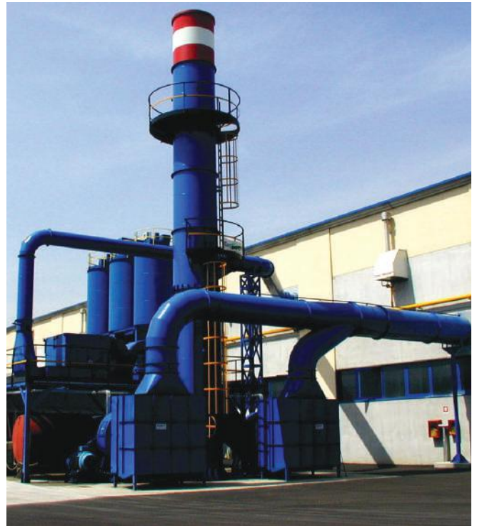
Centralized suction and filtration system ENERPROG - Italy
