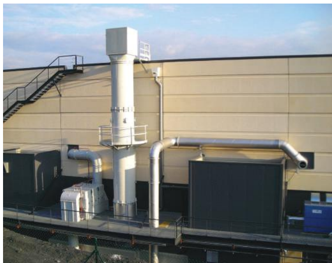
ENERPROG centralized suction and filtration system in number 2 modules for a total sucked flow of 32,000 m 3 /h dedicated to 4 presses - Spain
